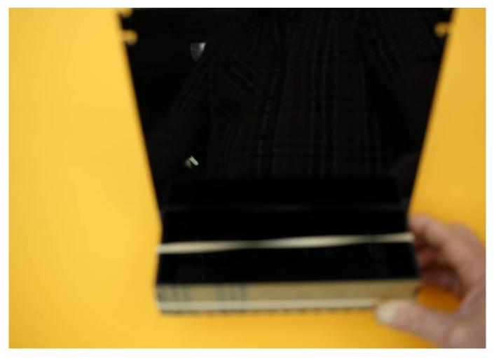
Dab glue into the joints, and fit the tank parts together. Do not worry about filling every joint with glue - water-tight sealing will happen later when silicone is applied.
