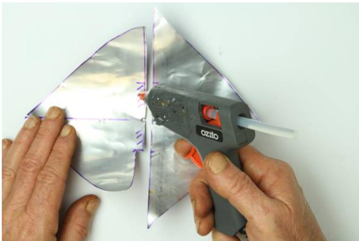
Use hot glue along the edge of the bottom piece to join the two halves together.
