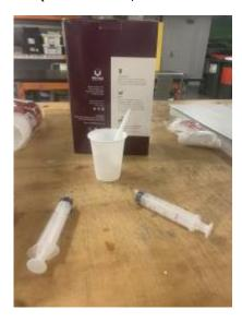
Again you need to workout what volume of the 2 Part Polyurethane Resin you need to mix up. Again you need to mix this thoroughly and you only have 2min "Pot time".
