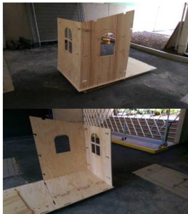
Then place the 3rd wall on one of the bases and and assemble using the corner joinery install roof truss using 70x30 pine (4 required). Repeat for the other base.
