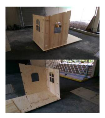
Then place the 3rd wall on one of the bases and and assemble using the corner joinery install roof truss using  $70 \times 30$  pine (4 required). Repeat for the other base.
