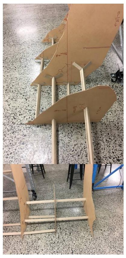
The support beams were pushed through the holes, and butted up to the adjacent Y-element. They were also located through holes in the next Y-element along to get them horizontal before gluing in place.
