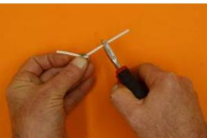
If it has not been done for you, separate the protruding wires (use a knife or cutters, or just pull them apart with your fingers).
